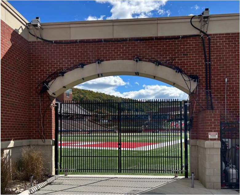
Field Entrance Gate (12' wide; 10'6" high)
